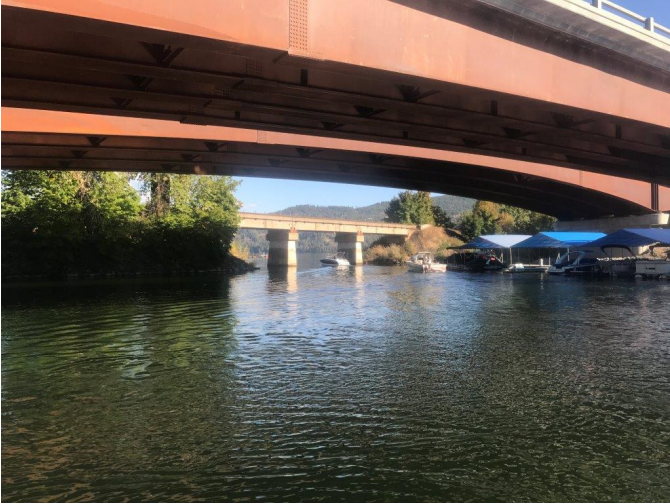
Photo 5: Bridge 3.1 – View of Bridge from the West side looking East
