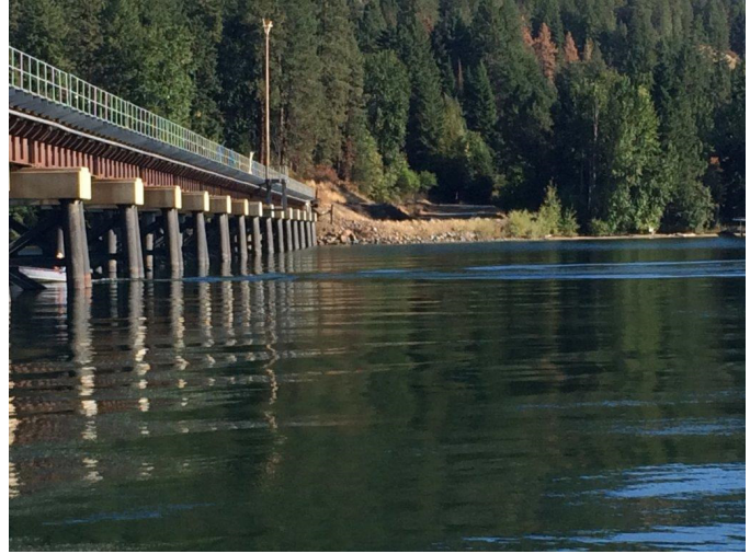
Photo 2: Bridge 3.9 – Close-up view of South end of Bridge
