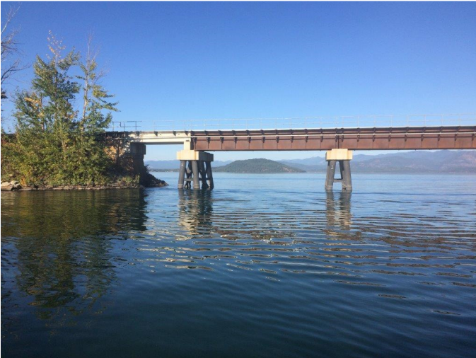
Photo 3: Bridge 3.9 – Close-up view of North end of Bridge
