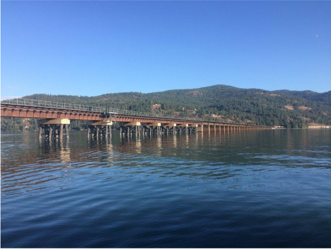
Photo 1: Bridge 3.9 – View of Bridge from West side looking Southeast
