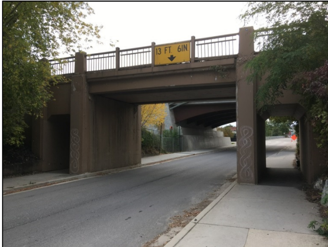
Photo 7: Bridge 3.0 – View of Bridge from West side looking East
