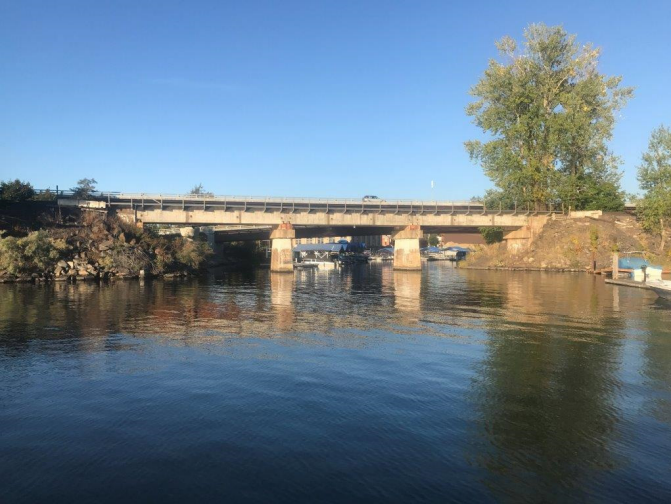
Photo 6: Bridge 3.1 – View of Bridge from East side looking West
