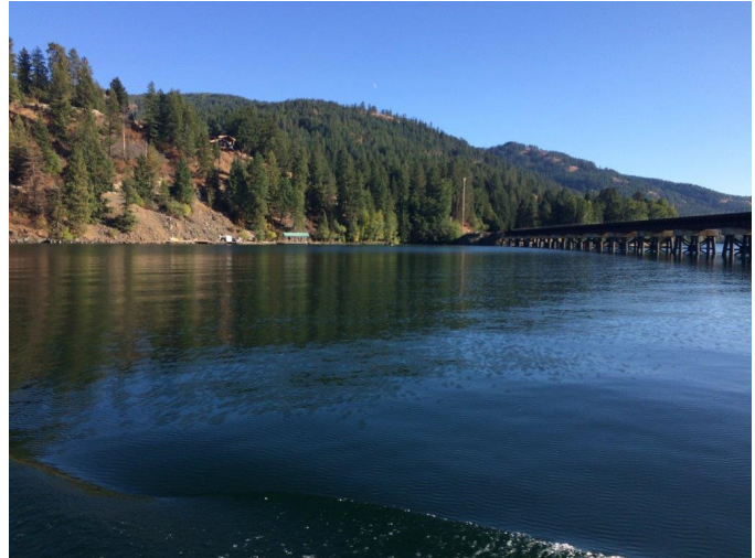
Photo 4: Bridge 3.9 – View of Bridge from East side looking South
